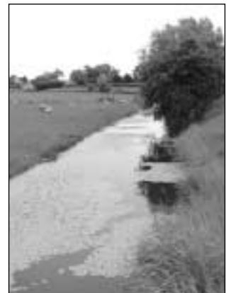
Engine Sewer, The Dowels
